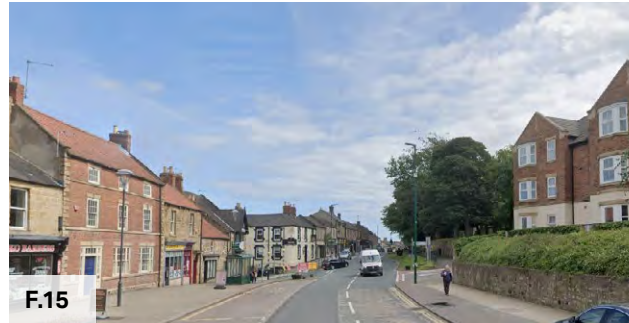
Figure 15: Apartments are elevated from the road to create a greater sense of enclosure at the eastern end of Front Street.
