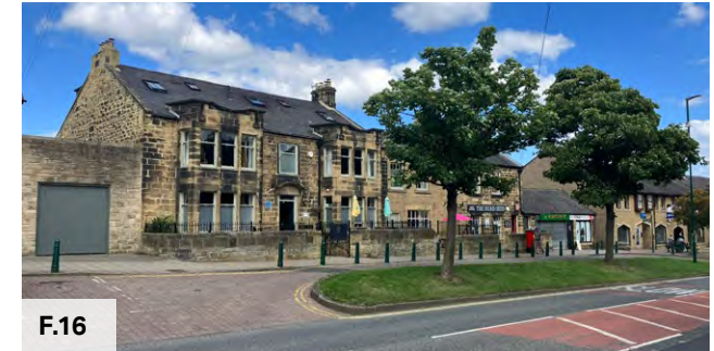
Figure 16: Lay-bys with mature trees are a feature at the western end of Front Street, creating large setbacks.
