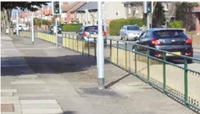
Freshly painted railing in West Bedlington Town Council Colours at West End School Bedlington.
